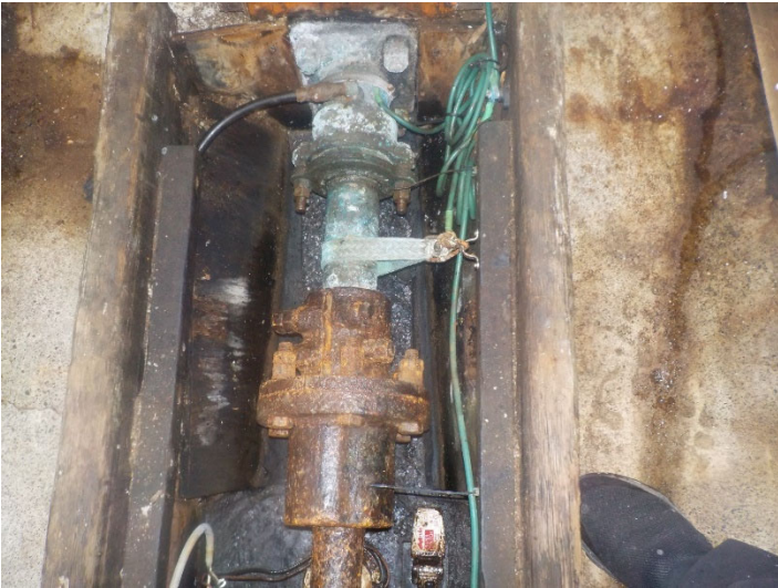
Figure 10 PACKING GLAND
